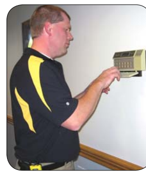
Dean Adams, District Energy Manager, checks the setting on a room thermostat as part of his efforts to track energy consumption.
